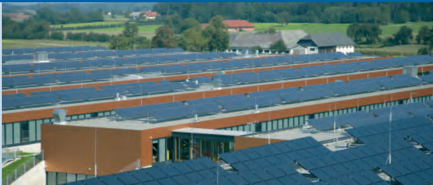
Fig. 1 - Currently the largest PV system in Austria is at Fronius company/Sattledt, 603 kW (photo Fa. Fronius).
