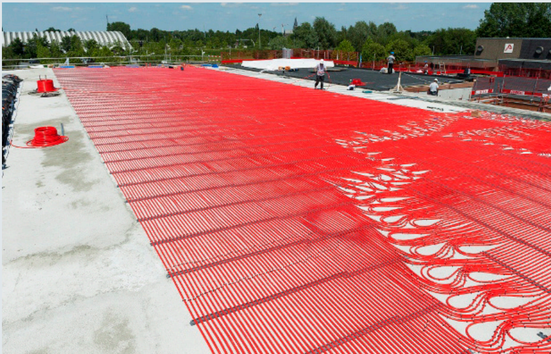
Figure 2. Build-up of the energy roof.
