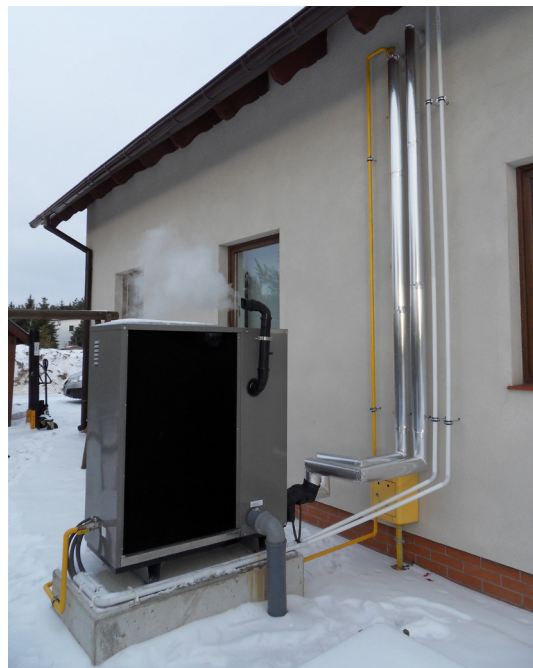
Figure 3. Gas driven heat pumps are tested with different climates and building types to find optimal configurations and system layouts.
