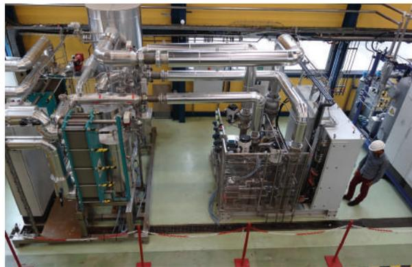
Heat Pump up to 140°C with water as working fluid.
