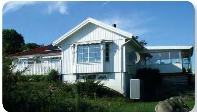
One of the studied buildings, located in Sweden. The building is equipped with an air-source heat pump and solar panels for DHW production.
