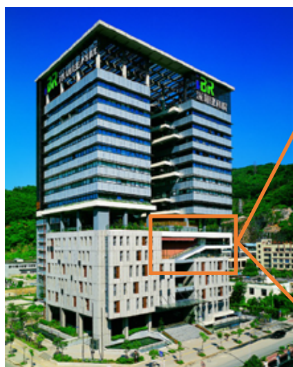
A typical mixed-mode building. The auditorium was designed with openable walls to make good use of natural ventilation. This space has achieved good thermal comfort and low energy consumption. Source: Shenzhen iBR, P.R. China
