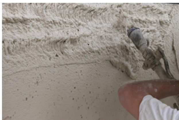
Application of Aerogel Mortar Rendering Source: EMPA
