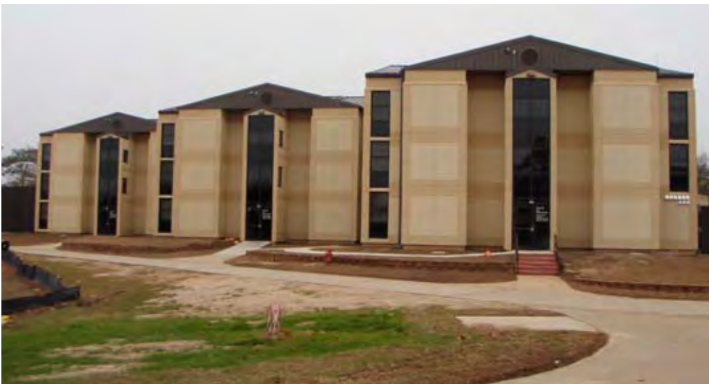
Renovation of barracks achieved a 45% energy use reduction through better insulation, improved airtightness, a dedicated outdoor air system, enclosed stairways with a vestibule and a covered atrium with increased usable space (Fort Polk, USA). Source: U.S. Army Corps of Engineers
