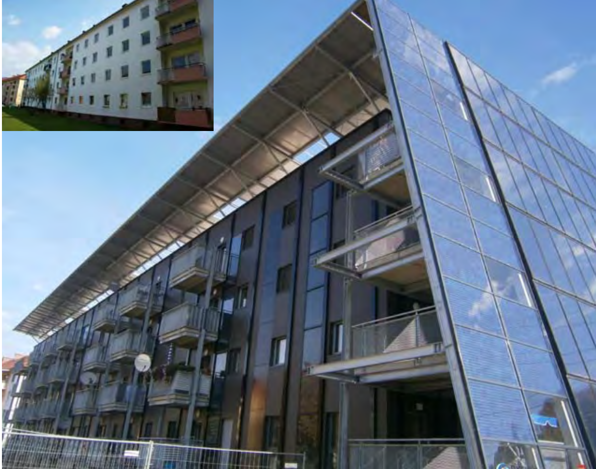
Ongoing EBC research into cost effective renovation: Kapfenberg case study – View of the existing (inset) and the renovated building (main picture). Source: AEE – Institute for Sustainable Technologies.
