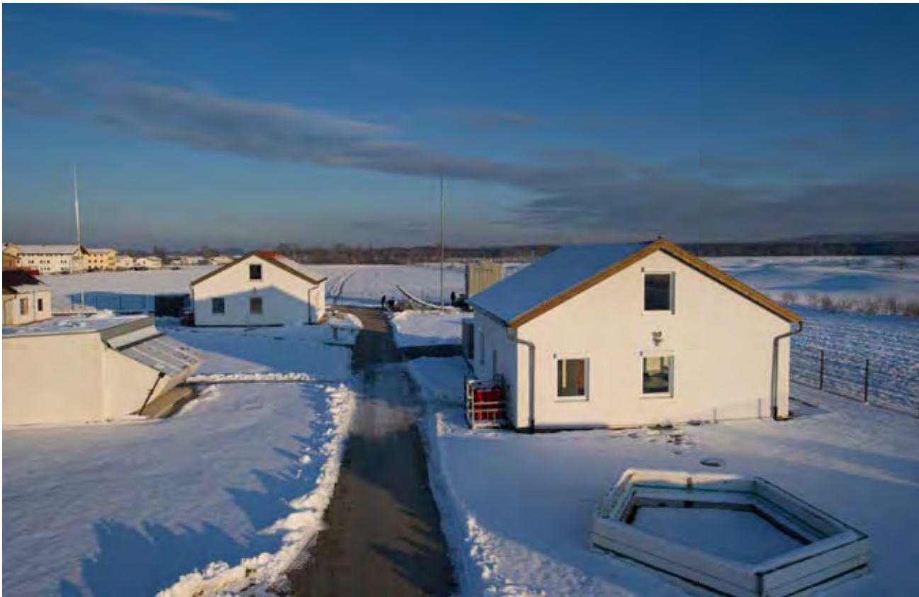
Detailed and well-documented full scale experiment in the twin test houses at Fraunhofer IBP, Holzkirchen performed in the project to validate common building energy simulation models and to develop 'grey box' models for the thermal characterization of buildings. Source: Fraunhofer IBP
