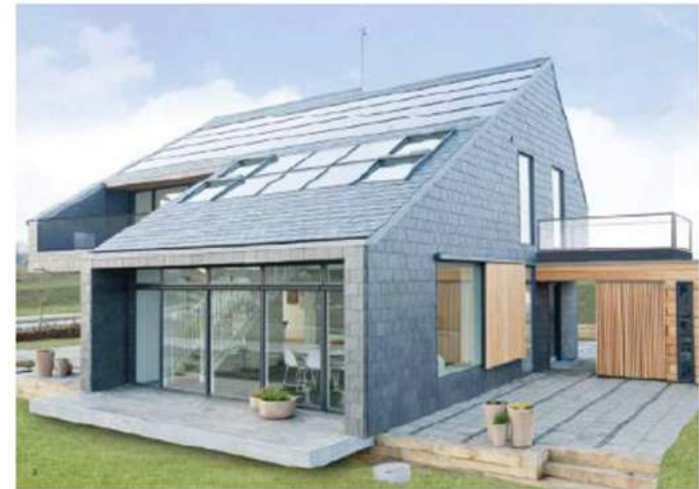
Fig. 1 South East view of the building
