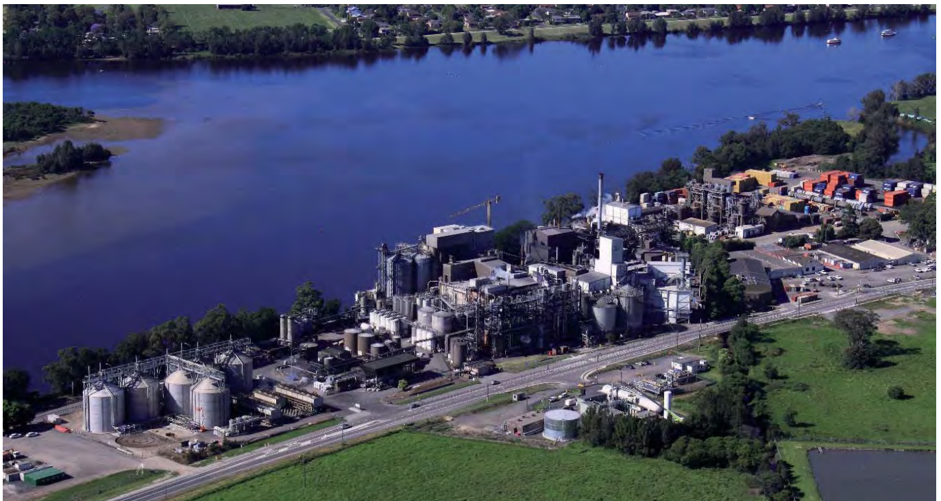
Figure 14. Bomaderry Plant, New South Wales, Australia (Dec 2011) [Manildra Group]
