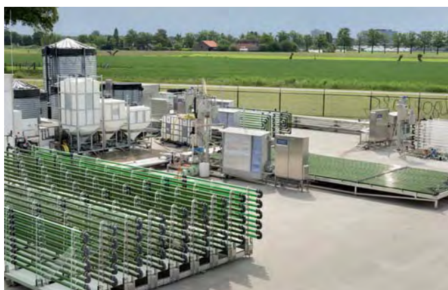
Figure 31. AlgaePARC Pilot Facility [Wageningen UR]
