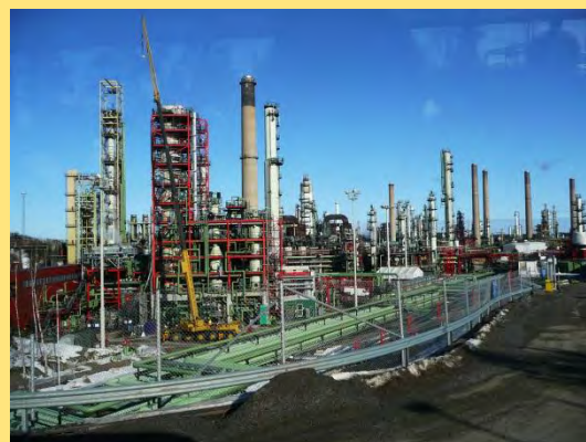
Neste Oil Refinery, Povo, Finland (Photo D.N. Bird)
