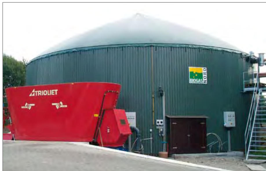
Photo 1: Anaerobic Digestion plant in Germany
