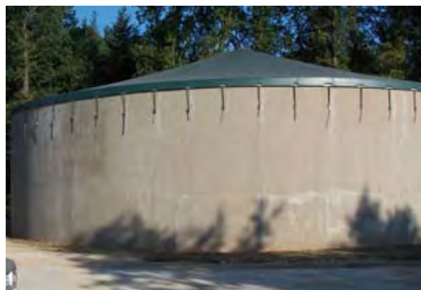
Photo 5: Covered digestate storage tank
