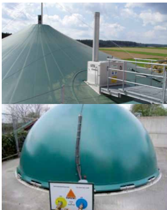
Figure 8 Gas storage in a flexible roof (top) and in a double membrane gas holder (bottom) (Photos: B.Drosg (top); A. Bywater (bottom))
