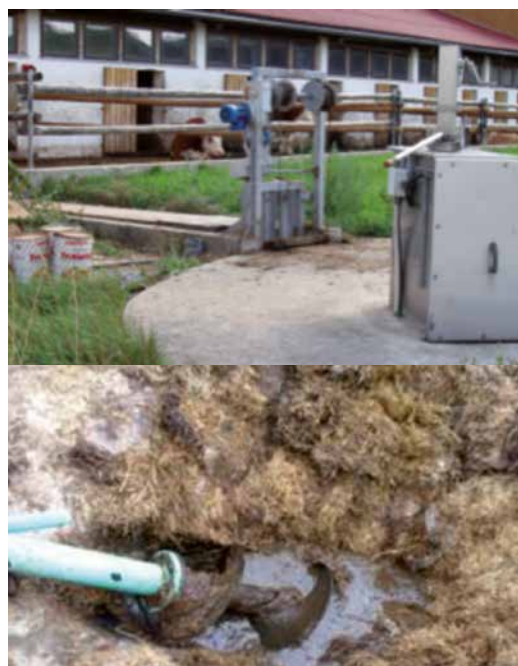
Figure 7 Digester feeding options; Gravity feed of manure into the tank – top photo: S. Baumann; Feedstock augered directly into a digester – bottom photo: A Bywater
