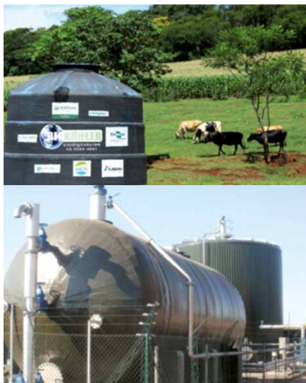
Figure 5 Upflow (top picture) and plug (lower picture) flow examples of digesters (Photo: Top: ITAIPU Binacional, Brazil; Bottom: Marches Biogas)
