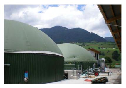
Figure 13: Biogas plant in Kägiswil, producing annually 1.5 GWh electricity and 1.7 GWh heat.
