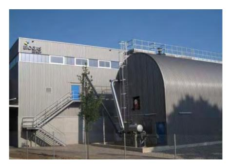
Figure 14: Thermophilic biowaste reactor of Biogas Zürich (© Biogas Zürich)
