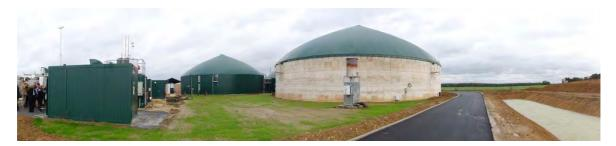
Figure 6: Biogas unit in Chaumes en Brie, France, owned by Bioénergie de la Brie Co. The plant produces biomethane and various products from agro food biowastes and manures. The biomethane is injected into the natural gas grid and feeds 5 cities located close to the unit.
