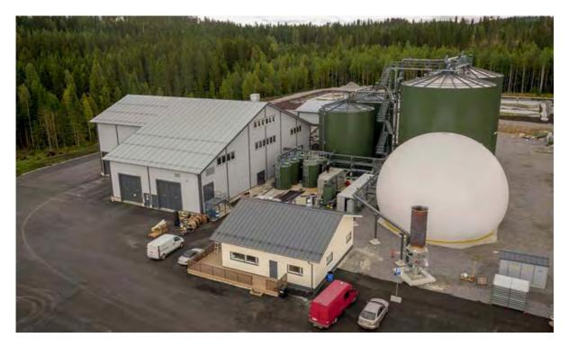
Figure 5: Biogas plant in starting phase in Kuopio. The plant has capacity of 60,000 tonne/year of sewage sludge, source separated biowaste, biowaste from grocery stores and supermarkets, and food industry wastes. Biogas production is about 34 GWh / year, and the biogas is delivered through a 5 km pipeline to Kuopio Energy that produces heat and electricity for Kuopio city.
