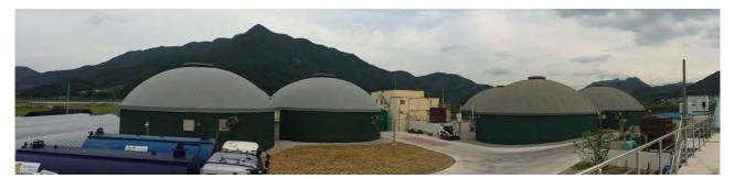
Figure 11: Yangsan Biogas Power Plant that is producing 1.0 GWh electricity (with 2.3 million Nm<sup>3</sup> biogas) annually. (source : Kyungnam Province, Korea)
