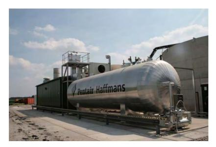
Figure 16: The biogas upgrading unit producing both biomethane and carbon dioxide at the Ecofuel biogas plant
