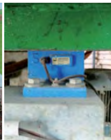
Figure 4 Weighing cell below the feedstock loading unit documents the mass input of feedstock to the digester
