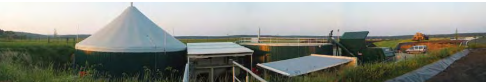
Photo 13: General view of a two-step, 500 kW e only energy crop digestion plant with digester 1 and dosing unit (center), digester 2 with integrated gas holder (left), silage clamps (background) and storage lagoon for the digestate (foreground right).
