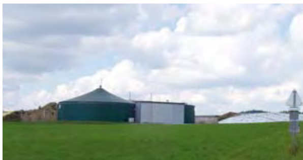
Photo 12: General view of a 2-step crop digestion plant with digester 1 and digester 2 combined with membrane gas collector. The silage clamp can be seen on the right.
