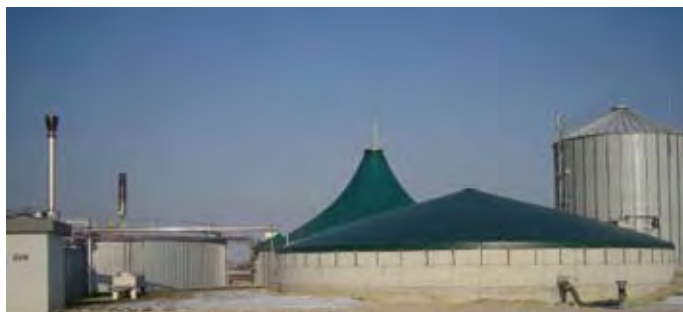
Photo 14 : General view of a 1 MW e crop co-digestion plant using two parallel digesters (left background) and a covered final digestate storage tank (centre foreground). Gas storage is integrated in digester 2 (background) and in the final storage tank (foreground), further storage capacity is provided in a dry gas storage tank (background right).
