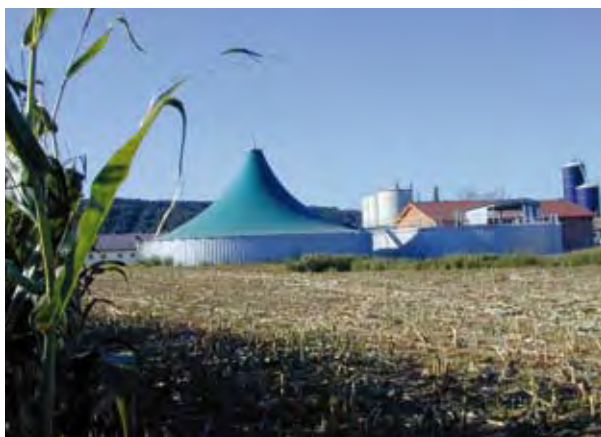
Photo 11: General view of a 2-step crop digestion plant with digester 1 (right) and combined gas collector and digester 2 (left)
