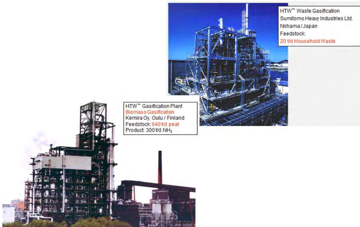
Figure 12: HTW Gasification plants in Japan and Finland
