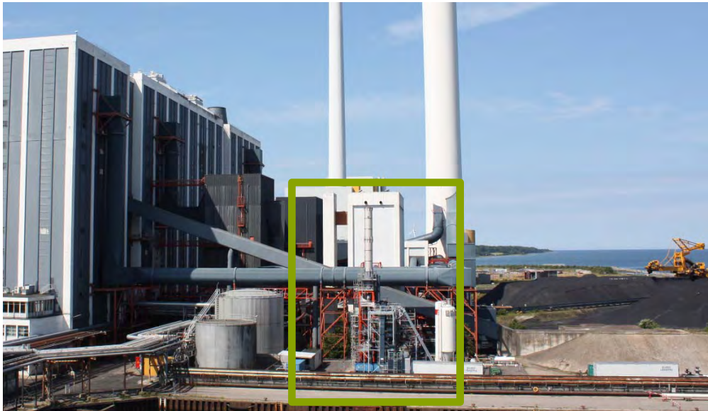
Figure 4: 6 MW demo plant
