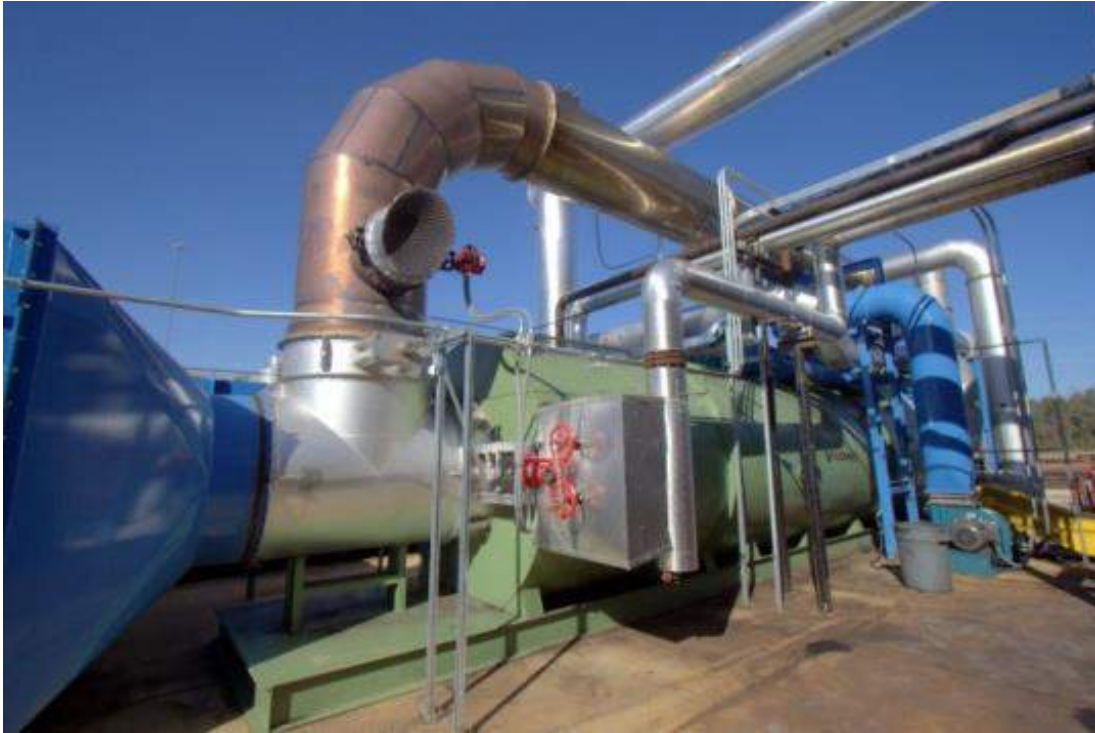
Figure 4-6 One of the hot oil systems at the Solvay Biomass Energy plant
