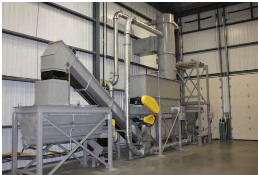
Figure 7.3 Predrying system and feeding bin of the Airex installation.
