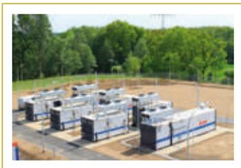
Fig. 9. 2MW Power to Gas unit based on alkaline electrolysis in Falkenhagen, Germany. The hydrogen is injected into the gas grid without methanation. (Source: E.ON)
