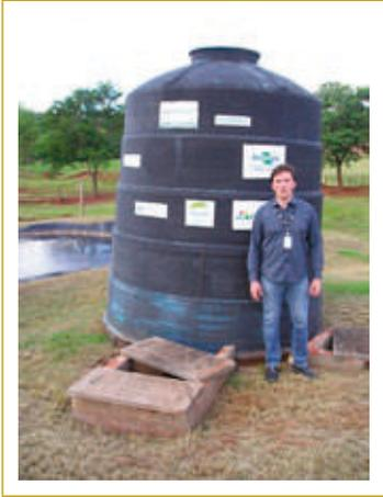
Fig. 4. Picture of one of 33 small scale (10 m<sup>3</sup>) digesters on 33 small family farms in Parana State in Brazil
