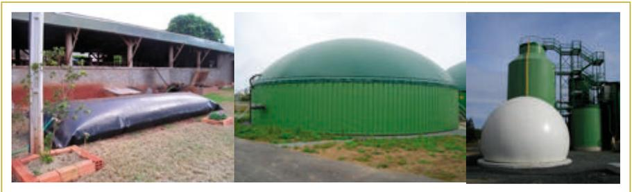
Fig. 7. Examples of biogas storage facilities: (left) a simple inflatable bag store on a very small farm; (middle) a flexible cover integrated into a digester; (right) a separate on-site gas store.
