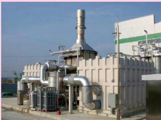
Figure 8 FCE's 2.8MW DFC3000 installed in Korea
