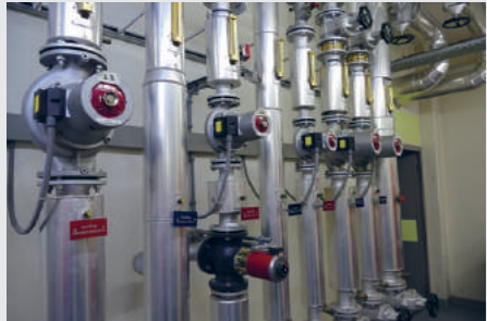
Five circulators. One circulator is a complete Motor Driven Unit consisting of VFD, motor, pump (Source: Impact Energy, 2016)
