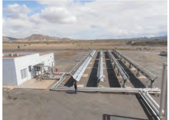
▲ Figure 6. View of a parabolic trough solar field for process heat (water desalination) at the Plataforma Solar de Almería.
