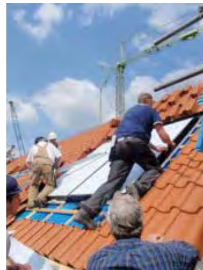
▲ Installing a typical Dutch roof integrated solar collector.
