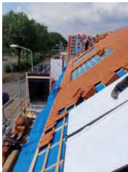
▲ Installing a typical Dutch roof integrated solar collector.
