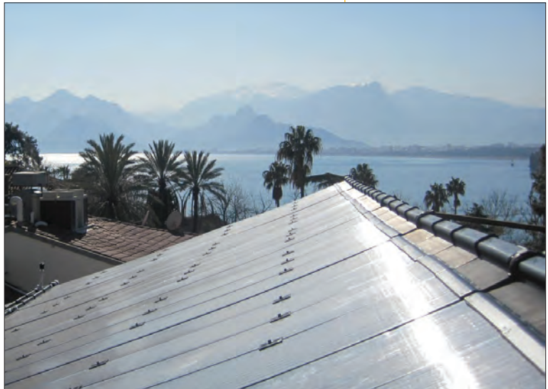
▲ Figure 1. Large domestic hot water system using polymeric collectors. Source: Magen Eco-Energy.
