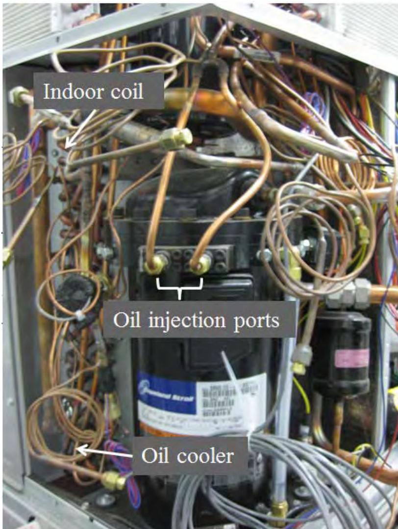
Annex 41: Oil-flooded compressor heat pump cycle concept to approach isothermal compression – schematic (above) and test system at Purdue Herrick Laboratories (below).
