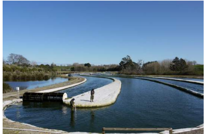
Figure 4. NIWA's demonstration-scale high rate algal pond system at Cambridge.
