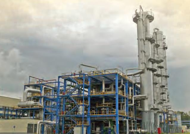
Bioethanol production from grain: 240,000 t/a plant operated by Agrana Bioethanol GmbH in Pischelsdorf near Vienna, Austria. Courtesy: Agrana.
