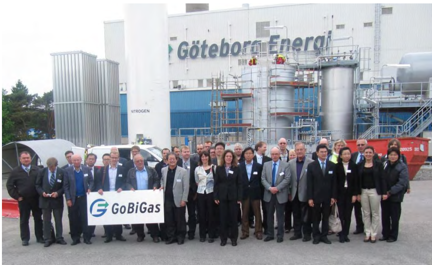
Visit to the GoBiGas biomethane production facility (under construction) during AMF ExCo 45
