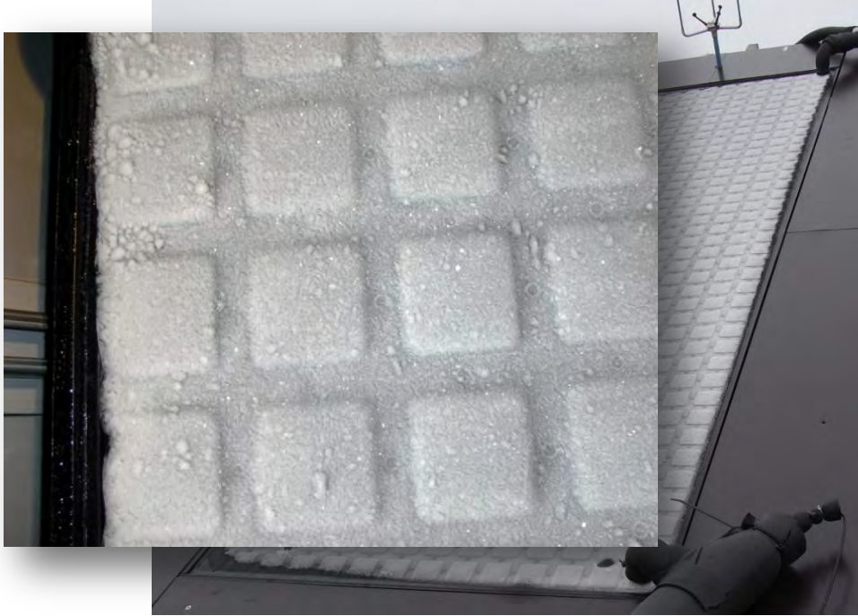
Figure 8: Frost on an uncovered solar collector operated below the dew point (source: Institut für Solartechnik SPF).
