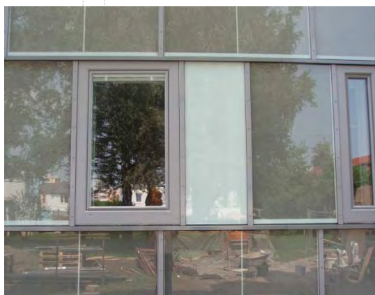
Figure 13: Window with integrated shading device and opaque field beside the window – covering supply and exhaust air ducts for ventilation
