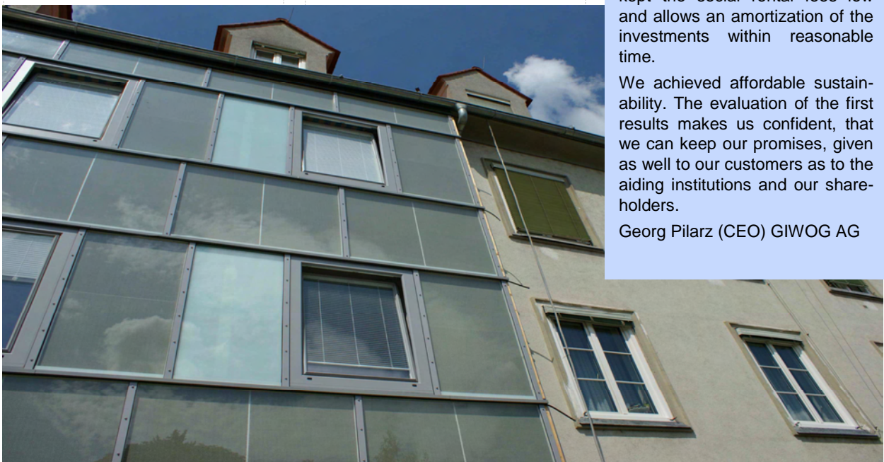
Figure 25: View on a renovated part (left) and a former part of the façade (right)
