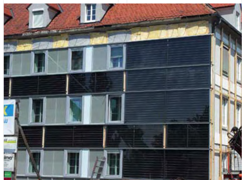
Figures 20-22: Sequence of assembly of the modules on the south-oriented façade.
