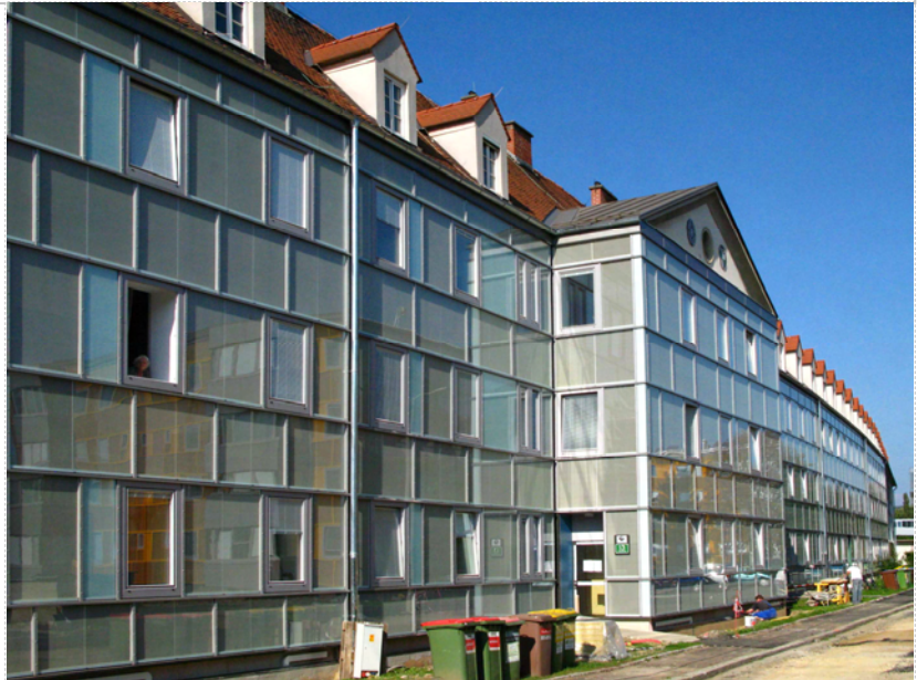
Figure 4: Dieselweg 13 and 15 – covered with new façade modules
