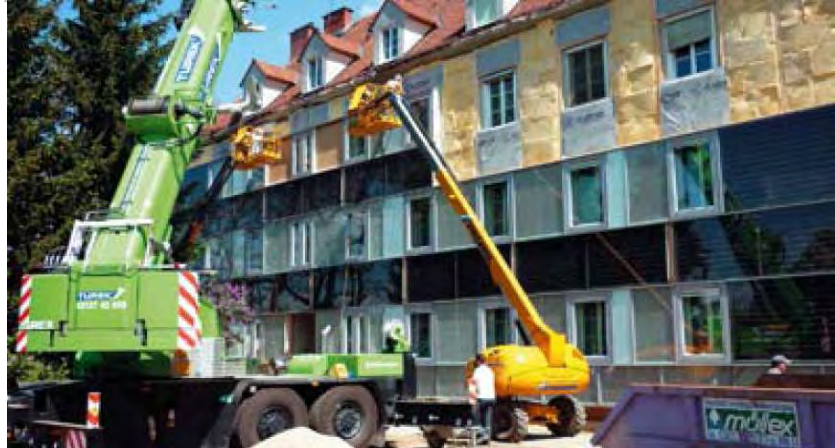
Figure 18: The preparation on-site is done by levelling laths. In-between the dissipation system and supply pipes are installed
