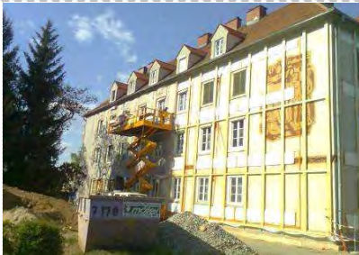
Figure 18: The preparation on-site is done by levelling laths. In-between the dissipation system and supply pipes are installed
