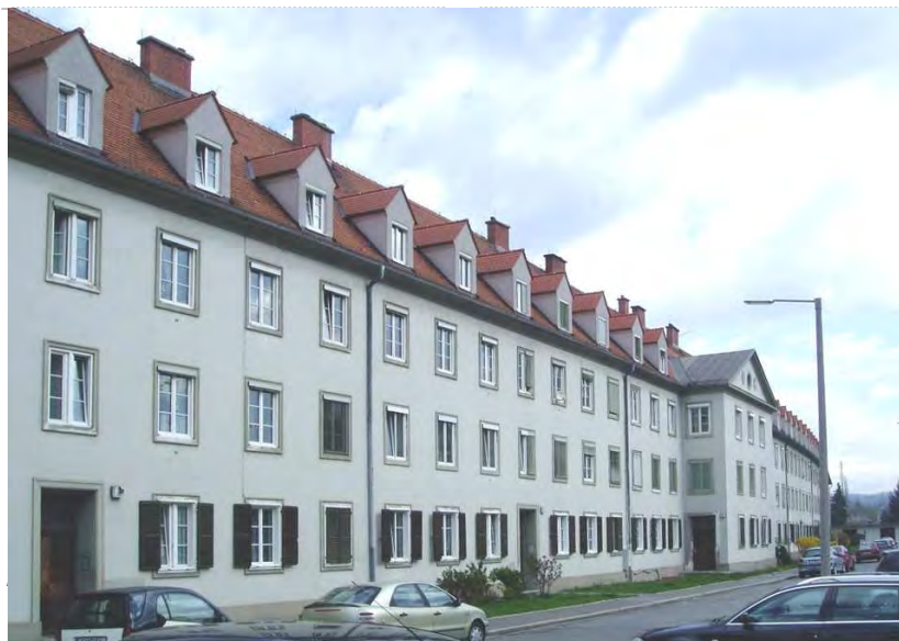
Figure 1: View of “Dieselweg 3-19”
