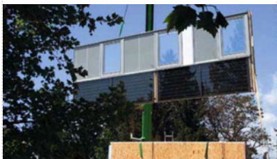
Figure 19: The solar collectors were integrated into the pre-fabricated modules
