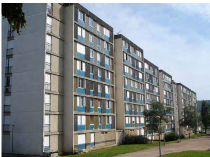
Figure 31: Test building for RECOLCI façade
