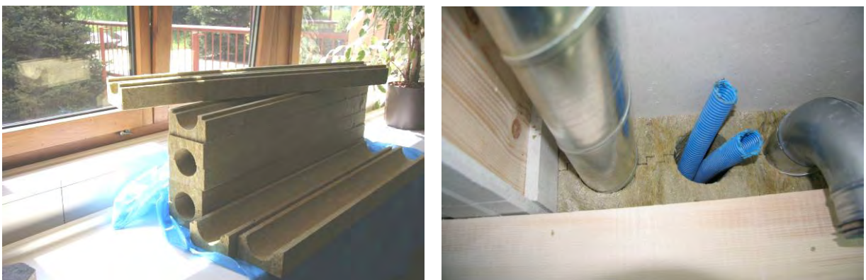
Figure 17: sectional insulation for ventilation ducts (Flumroc, Switzerland)
