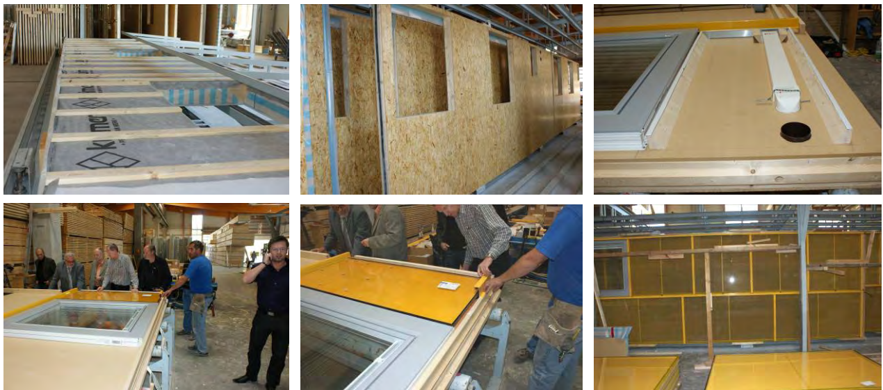
Figure 3: Assembling the prototype in the fabrication of carpentry Kulmer Bau (Source: AEE INTEC)
