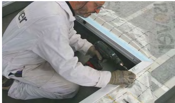
Figure 18: First insulation layer
