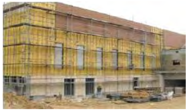
Figure 18: First insulation layer
