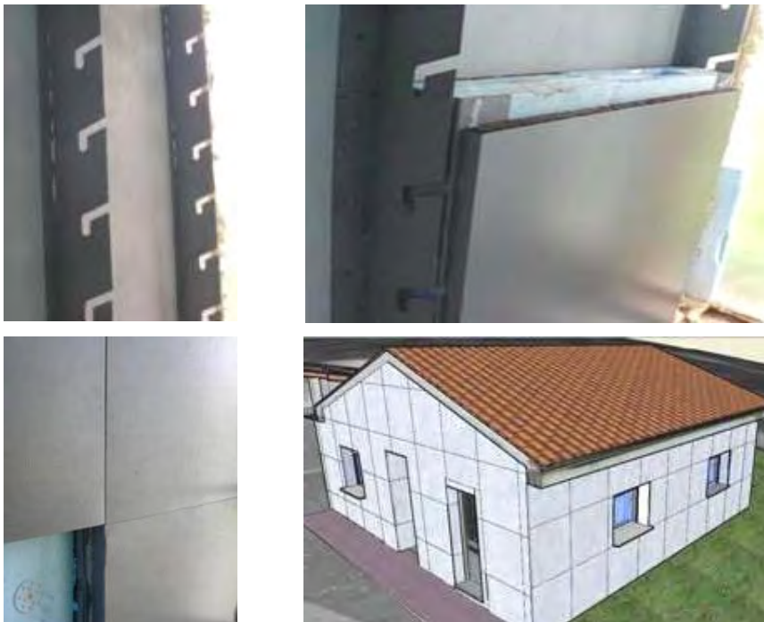
Figure 10: Steps needed to apply the retrofit module to the case study building
