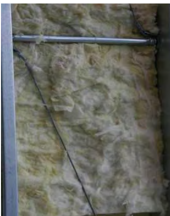
Figure 20: Insulation between two adjacent modules
