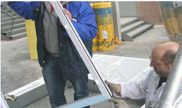
Figure 19: Mounting of windows
