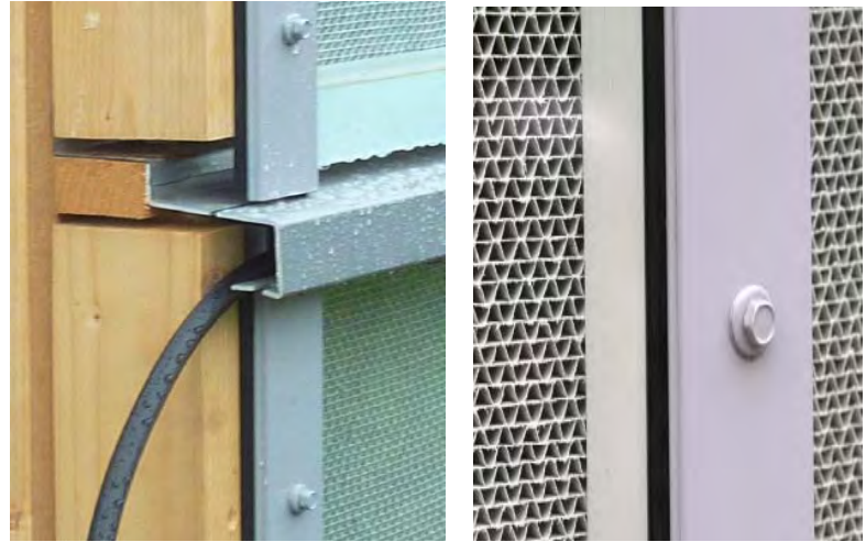
Figure 11: The upper picture shows the vertical joints with the cover strips fixed by screws. The picture below shows the horizontally mounted façade plate to ensure the sealing against driving rain (Source: gap-solution GmbH)
