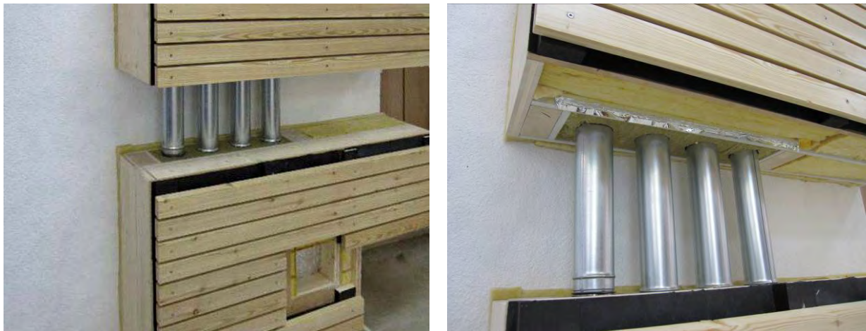
Figure 19: Model at Swissbau 2010 construction trade fair (Bächi Holzbau). Here, the façade is designed with timber rainscreen cladding. F4.1 module with push-fitted ventilation ducts
