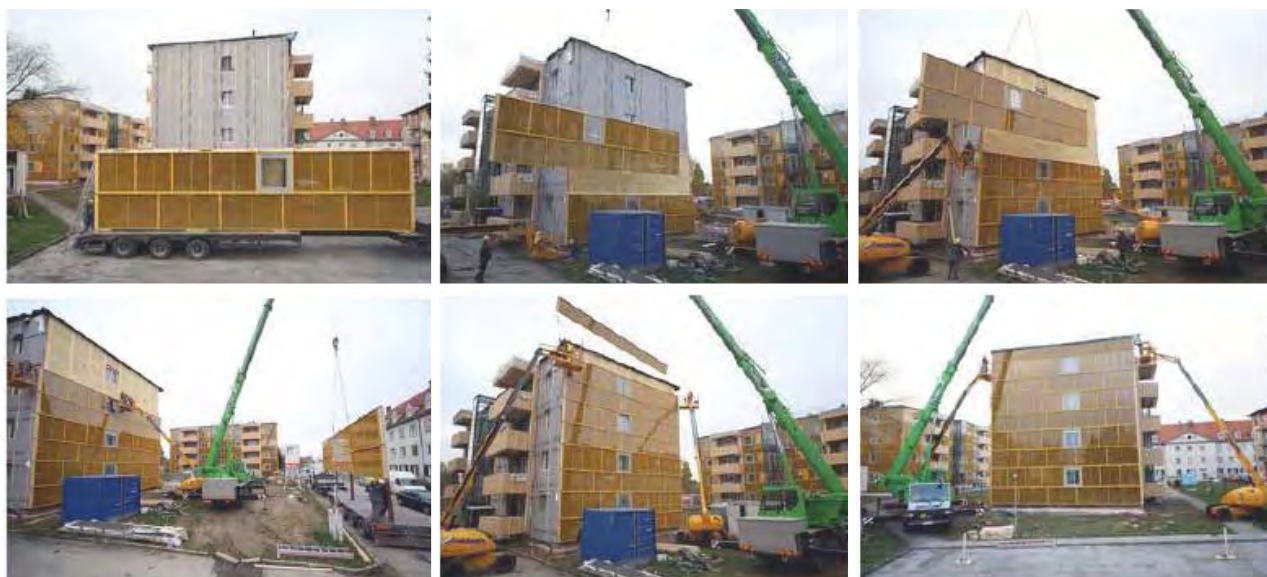
Figure 17: Transport on-site and assembling procedure (Source: gap-solution GmbH)
