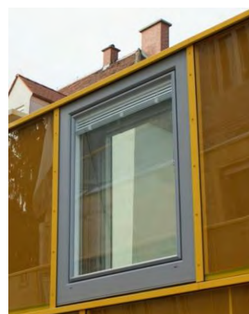
Figure 29: Blinds mounted "intermediate" (in-between the glass-panes) – to be used for plane façades.
