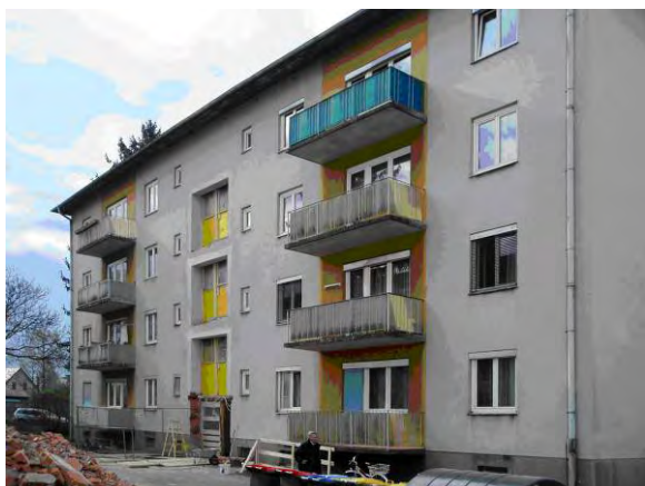
Figure 10: Balconies before renovation within residential area Dieselweg, Graz
