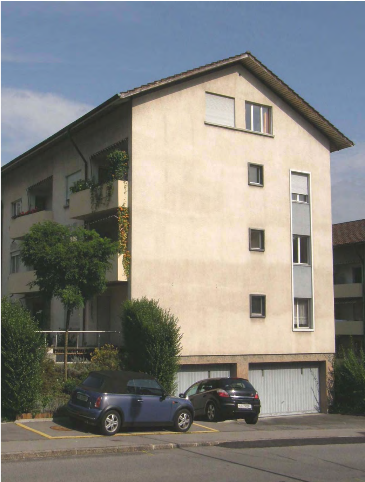
Northwest façade of case study building, Lucerne (see chapter 6.5), photo by R. Fischer, HSLU-CCTP
