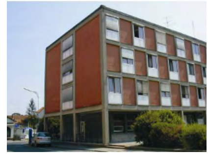
Figure 7: Building stock – skeleton construction (Source: LIG Steiermark)
