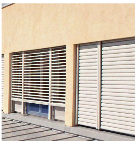
Figure 28: External venetian blinds - "all-metal". Very common used within object-range (robustness in case of wind-loads).
