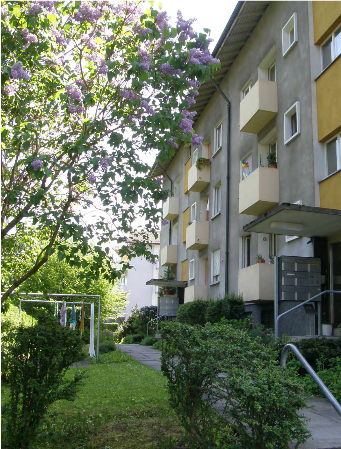
Northeast façade of case study building, Lucerne (see chapter 6.5), photo by R. Fischer, HSLU-CCTP
