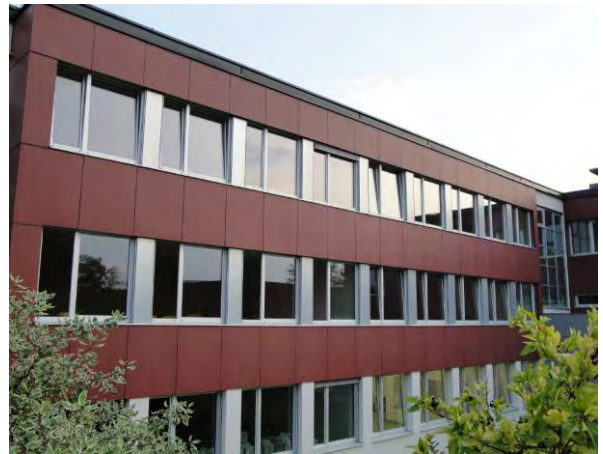
Figure 9: South-east oriented class-room windows – shaded with exterior blinds
