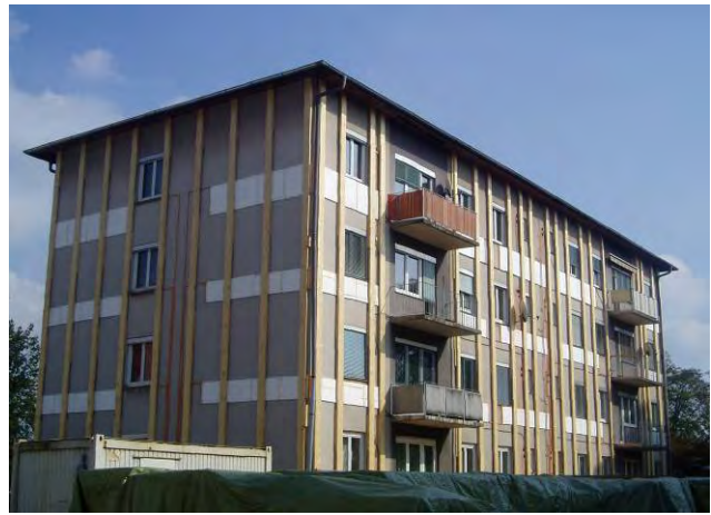
Figure 31: Levelling laths made of a timber substructure. Example: Dieselweg, Graz
