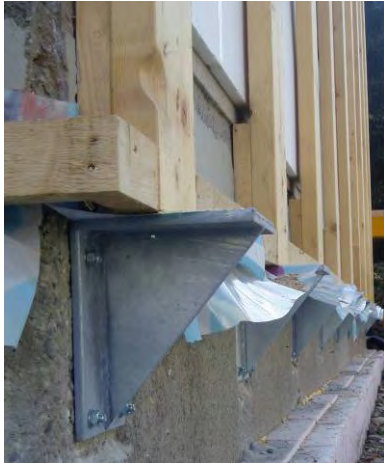
Figure 30: Steel angles as support brackets at the bottom. Example: Dieselweg Graz
