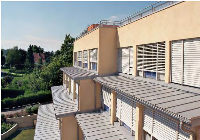
Figure 8: South-west oriented windows – shaded with exterior blinds (Source: Ziv. Ing. Büro Boder)
