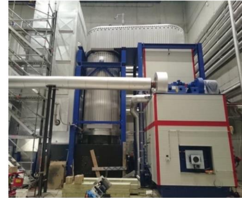
Figure 4. Boiler (KCO Kohlbach) with SNCR (ERC) (left) and electrostatic precipitator (Scheuch) (right).
