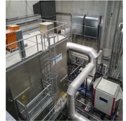
Figure 4. Boiler (KCO Kohlbach) with SNCR (ERC) (left) and electrostatic precipitator (Scheuch) (right).
