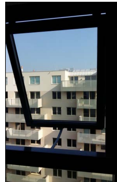
Extract ventilation unit and supply air window source: Peter Holzer
