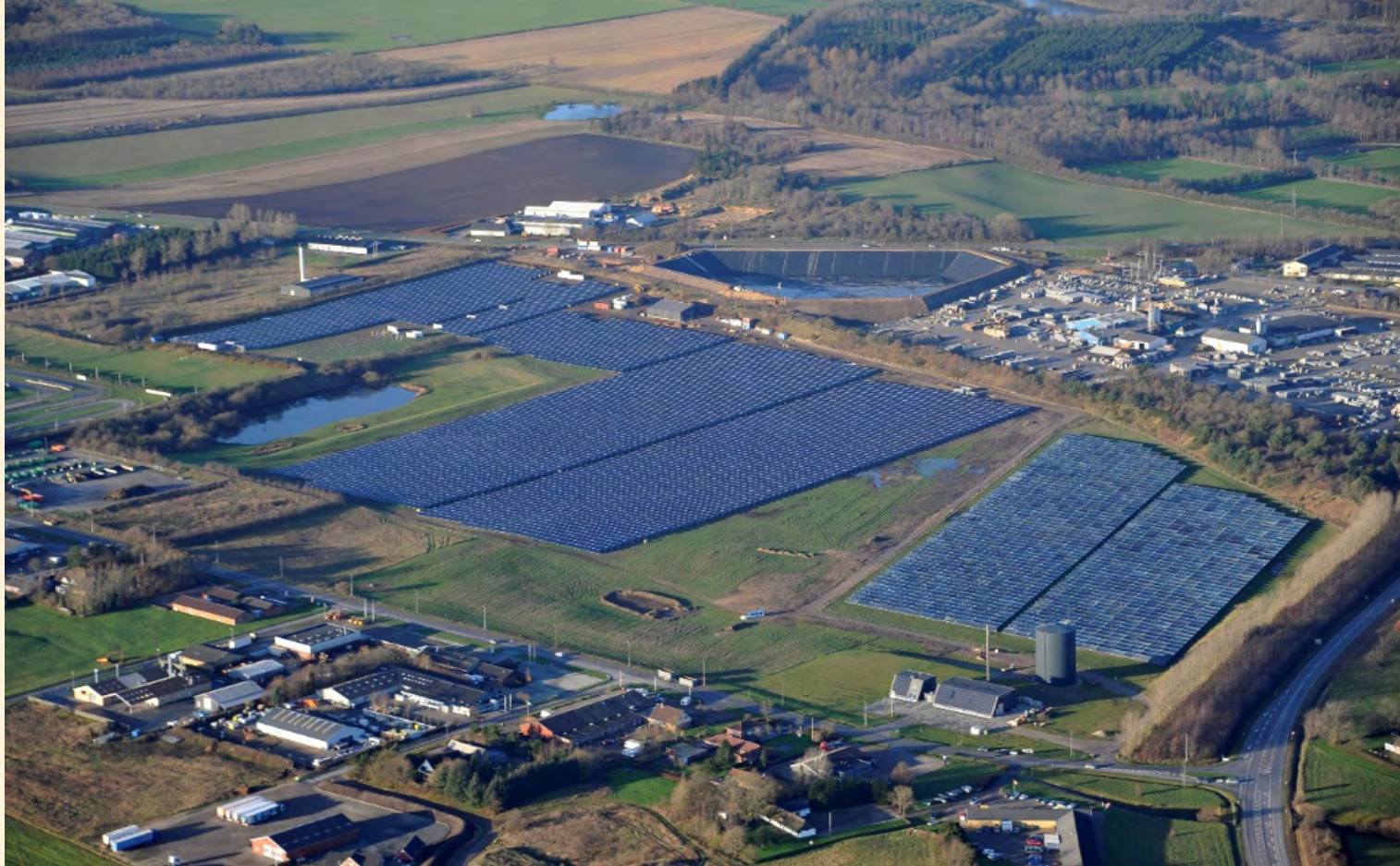
World Largest Solar District Heating Plant Vojens, DK, 70,000 m 2 (49 MW), 200,000 m 2 Source: http://www.vojensfjernvarme.dk
