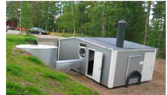
Bioenergy center Jyväskylä (Small-scale Combustion)
