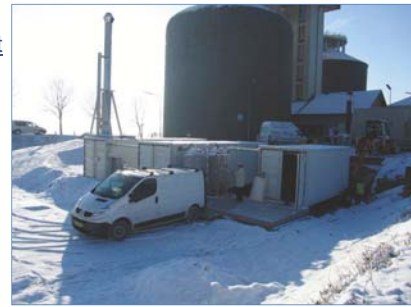
Construction site of upgrading plant in Wiener Neustadt (Lower Austria)
