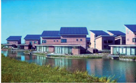
112 kWp integrated PV system, The Netherlands
