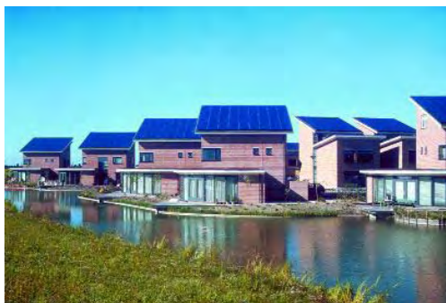
112 kWp integrated PV system, The Netherlands
