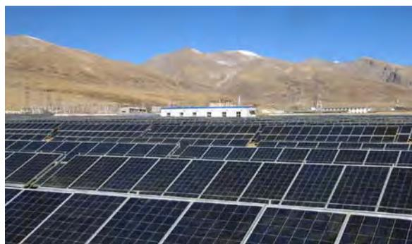
▲ A large-scale (10 MW) array of photovoltaic panels (YangBaJing, Tibet).
