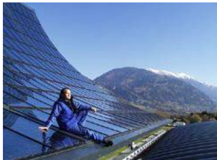
Figure 14: Solar Thermal Plant 23
