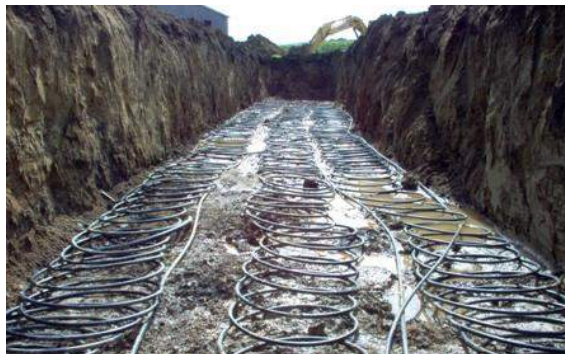
Figure 18: Geothermal Heat Pump - Horizontal Trenches 36
