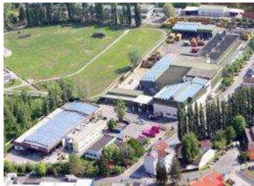
Figure 24: District heating plant/AEVG Graz - Austria 79
