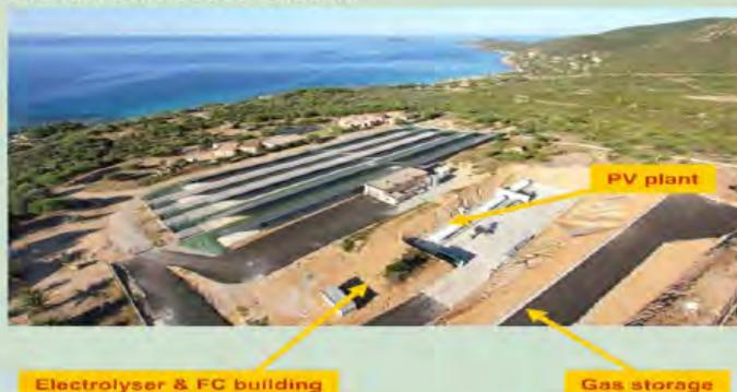
Smart grid technology is at the forefront of France's future for renewable hydrogen production and lean CO<sub>2</sub>. The Myrte platform, an experimental project that links a photovoltaic farm and hydrogen fuel cells system to an electrical grid connection, was inaugurated early in 2012. The objective is to control the system power output on the grid during critical hours of operation.
