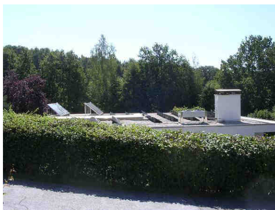
Figure 2 – single family house
