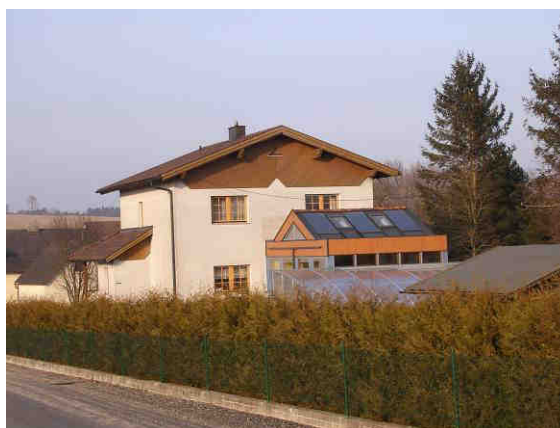
Figure 2 – single family house
