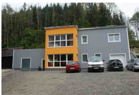
Figure 2 – single family house
