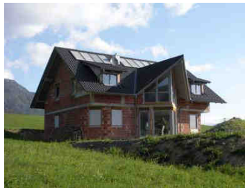
Figure 2 – single family house
