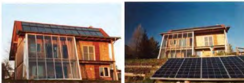
Figure 3-1: View of the private house "Jungreithmayr" with installed solar heating and cooling system (Source: SOLutiouon Solartechnik GmbH)
