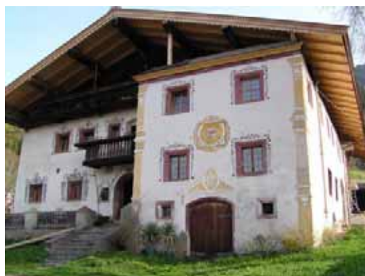
picture 5: Thermally renovated listed farmhouse with stone masonry in Kirchbichl / Tyrol
