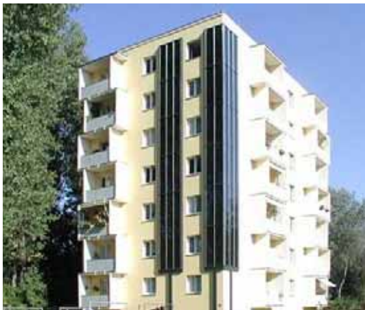
picture 19: Well designed integration of 90 m 2 of solar thermal panels into the building façade of the object 'Admonterstraße', Krems (image source: GEDESAG [7])
