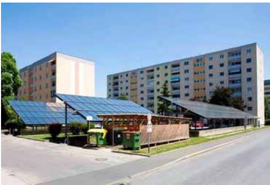
picture 28: Solar thermal collectors build as outdoor car roofing for an apartment building in Graz (Grottenhofstrasse), image source: ENW Ges.m.b.H. [31]
