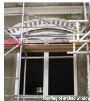
Roofing of arched window
