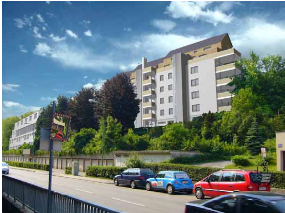
Broschüre 120: Apartment building in Kierling
