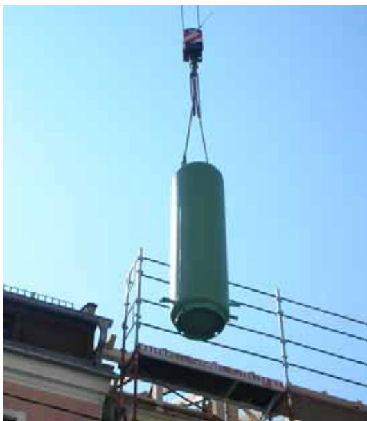
picture 33: Example for the emplacement of a standard water store for solar combisystems located in the old town of Graz, image source: Eduard Wasserfaller
