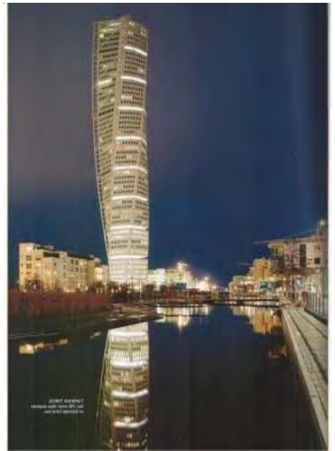
Turning Torso, an apartment building in Malmö, Sweden: all the corridors lit by LED lighting
