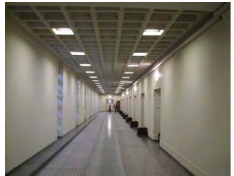
20 W tungsten halogen lamps above the doors replaced by 2 x 3 W LEDs
