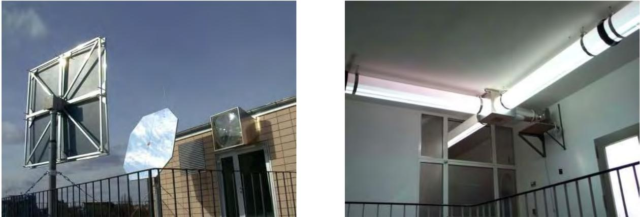
**Figure 5-29.** Pictures from an Artheliop project installation in Berlin. The heliostat on the roof supplies the light pipe with concentrated sunlight (left). An electric light source supplies the light pipes with electric light when needed (right).
