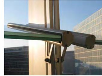
**Figure6-44.** Louvresinlightpenetration mode–110°slope.
