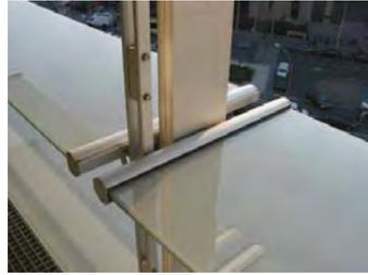
**Figure6-43 .** Louvresinhorizontalposition–90°slope. mode–110°slope.
