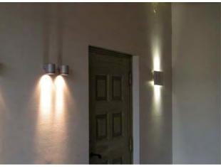
**Figure 10 - 36.** 2x35Wtungstenhalogenlampsreplaced by2x3WRebelLEDsgivinglightupanddown.
