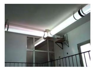
**Figure5-29.** Pictures from an Arthelio projectin stallation in Berlin. The heliostaton theroof supplies the light pipe with concentrated sunlight (left). An electrical light source supplies the light pipes with electrical light when needed (right).
