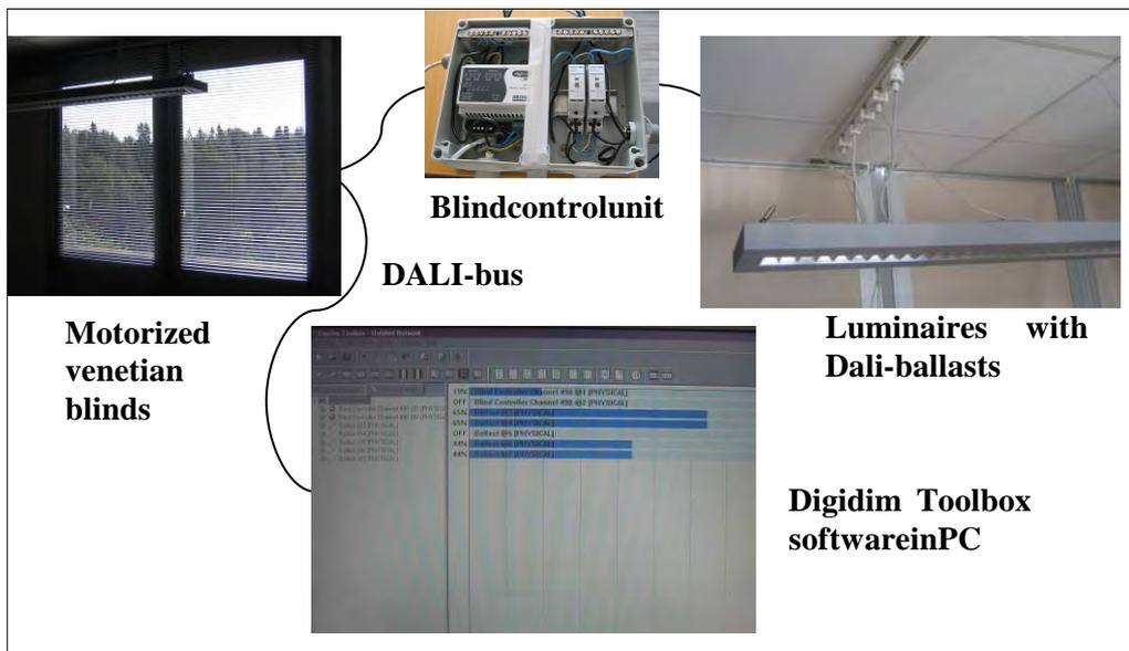
Figure 6-49. The integrated control system interfaced to DALI bus.
