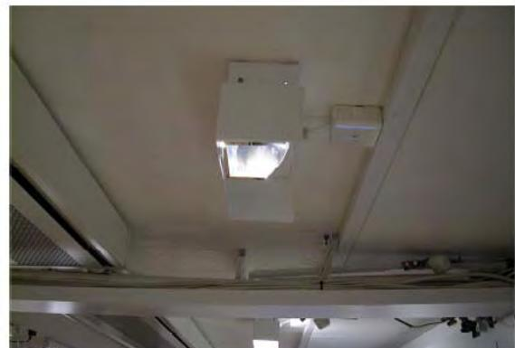
**Figure 10-31.** Lighting with Fortimo luminaire.
