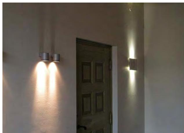
**Figure10 -36.** *2x35Wtungstenhalogenlampsreplaced by2x3WRebelLEDsgivinglightupanddown.*
