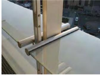
**Figure6-43 .** Louvres in horizontal position–90° slope.
