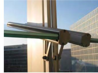
**Figure6-44.** Louvres in light penetration mode–110° slope.
