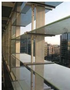
**Figure 6-37.** *Louvres in horizontal position.*
