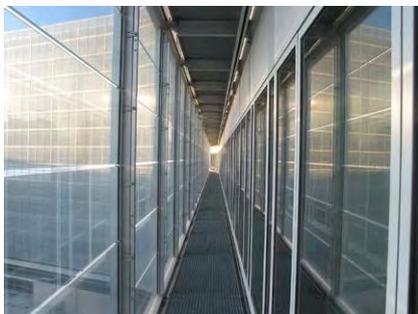
**Figure 6-36.** *View of the large cavity and the louvres in vertical position. horizontal position. December-14:00*
